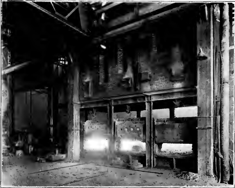
FIG. 108.—A. & W. Re-heating and Continuous Furnace.
